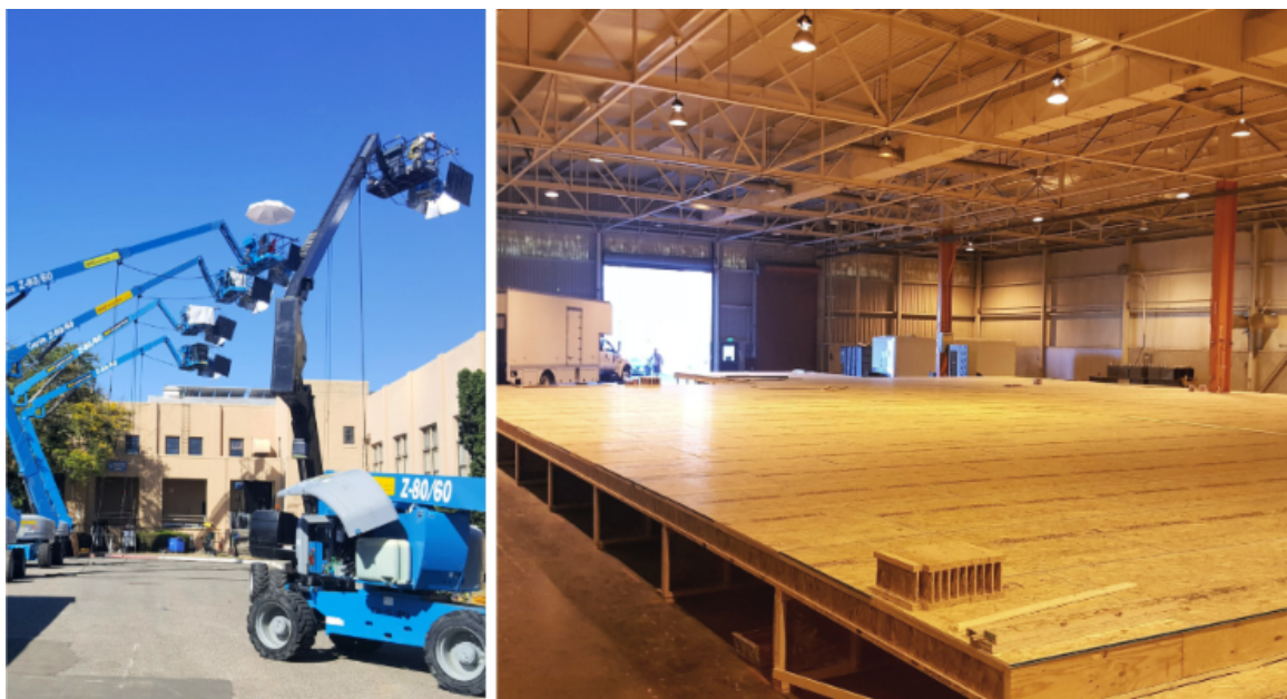
(left) A bevy of boom lifts is part of the equipment readily available on the island. (right) Historic Building 1310 was once used to build warship components, but now houses three sound stages totaling more than 115,000 square feet.
